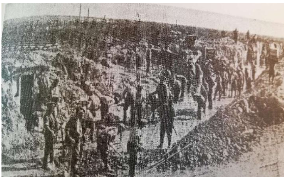
Photograph in A Private's War of the 5th Northamptonshire making roads (James, 2013, page 207).
