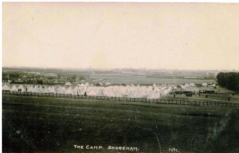
Shoreham Camp. By kind permission of Shoreham Fort Trustees.
