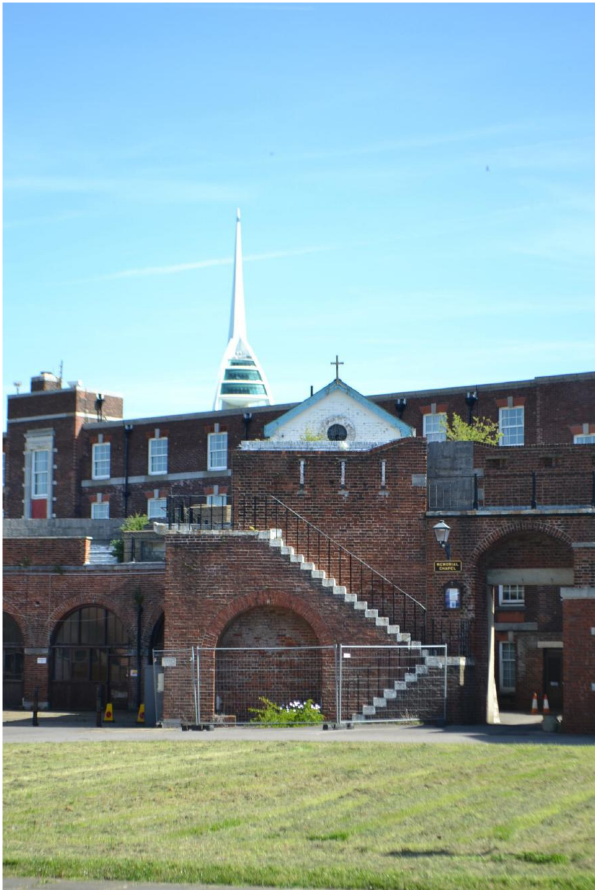
HM Submarine Chapel viewed from within Fort Blockhouse (Spinnaker Tower, Portsmouth in background)
